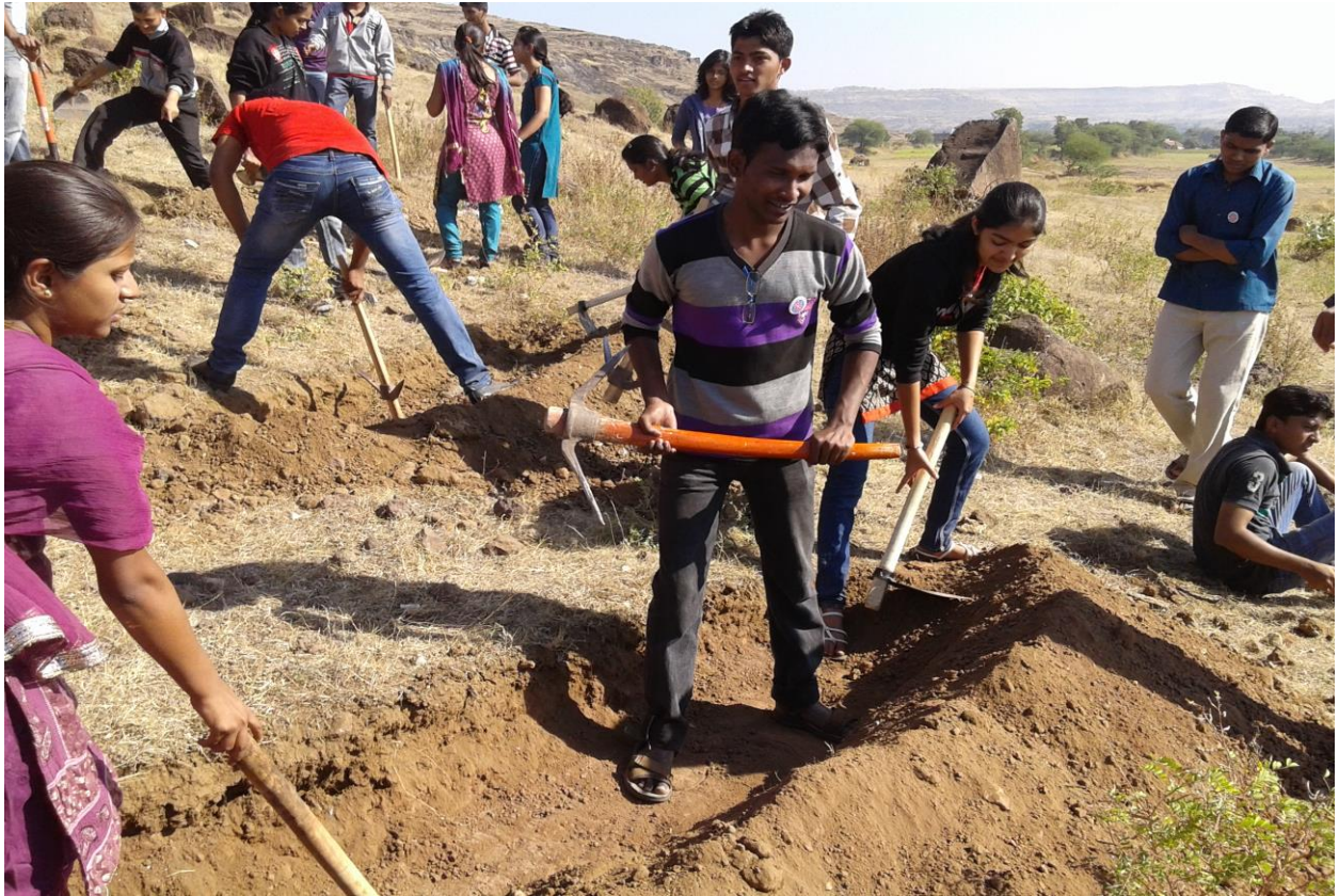
CCT construction at Sukewadi site
