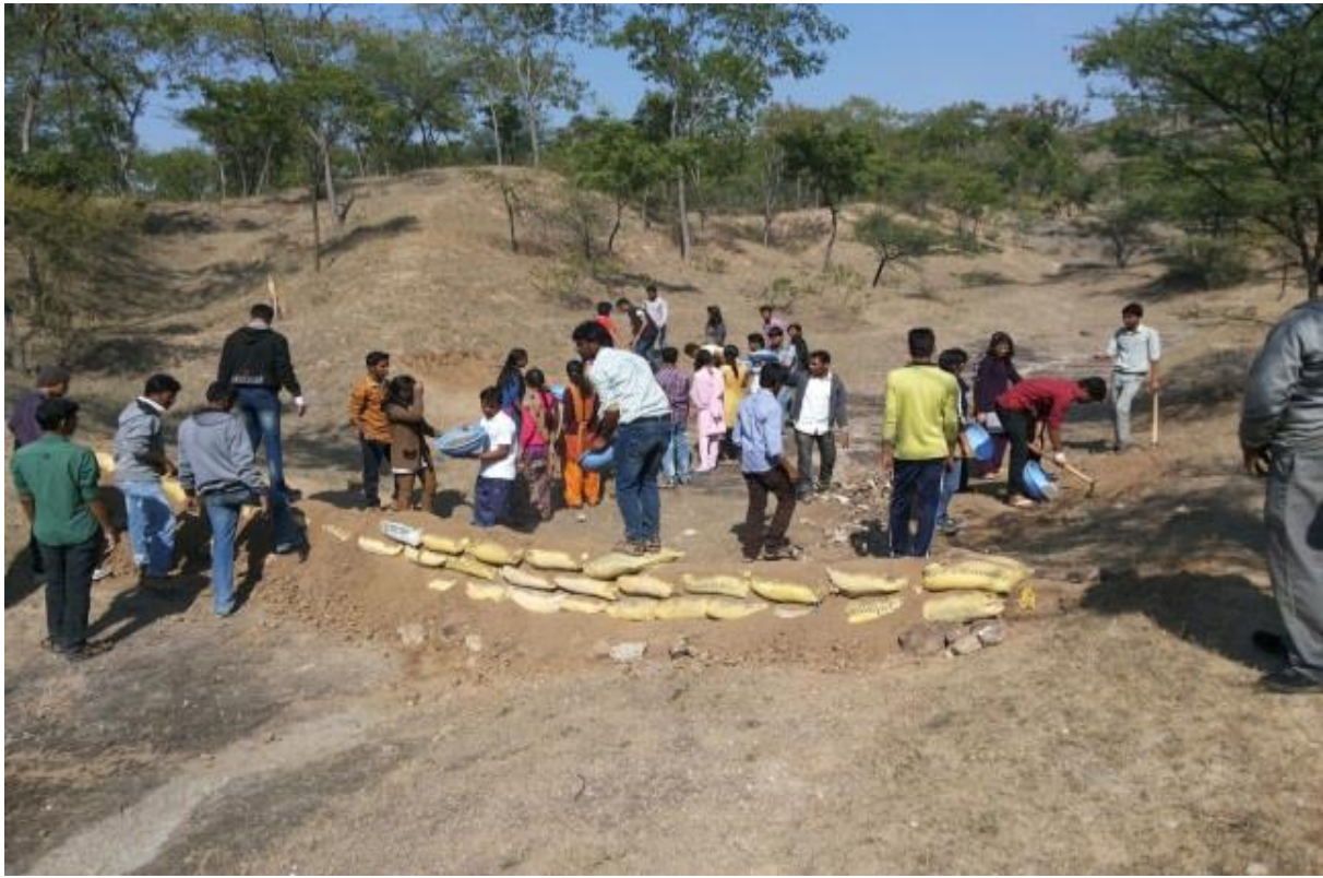
Students volunteers constructing the Water Canal at Sukewadi-Khanjapur
