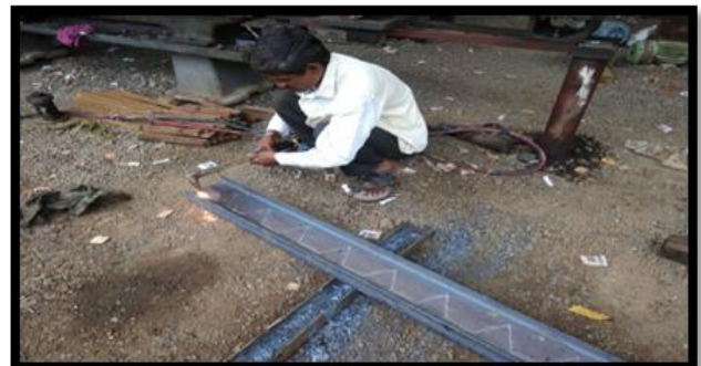
Fig. 5. Cutting of the beam
