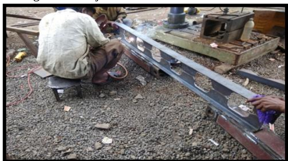
Fig. 7. Welding of Castellated Beam
