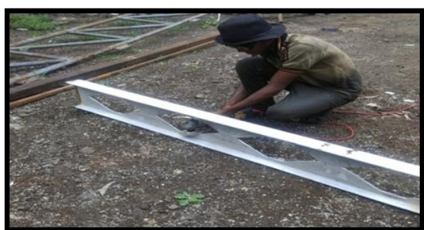
Fig 8. Grinding of a Castellated Beam
