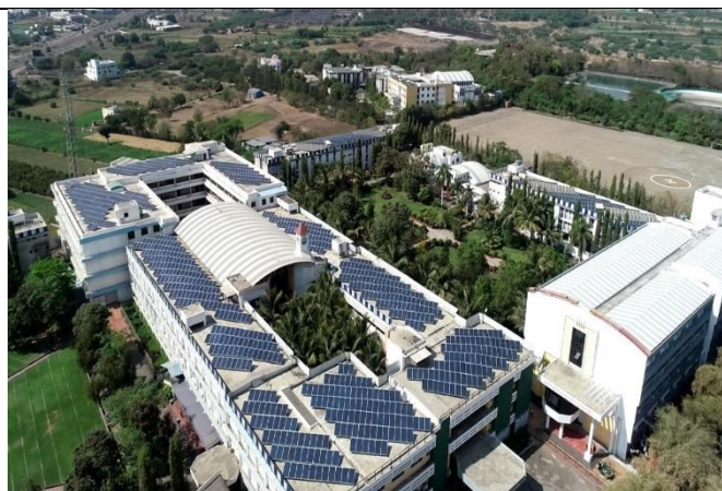
400KWp Roof top SPV System
