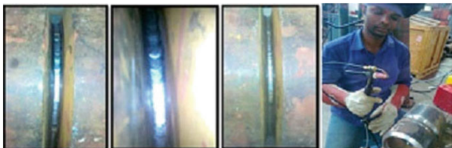
Fig. 8 Root pass welded by Tip TIG process (Santhakumari 2018)
