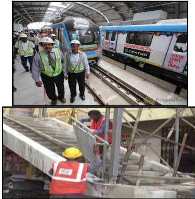
Fig.6: Hyderabad metro corridor II
