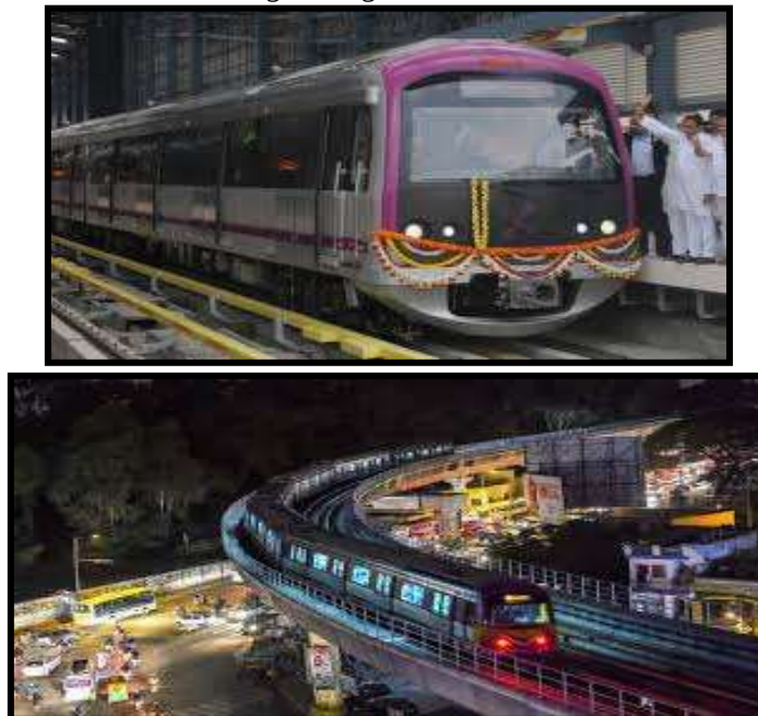
Fig.10: Bengaluru metro project Source: thehindubusinessline.com
